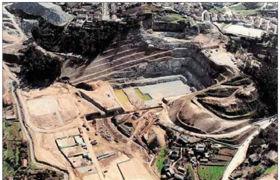
Fig. 3: General View of the excavation
