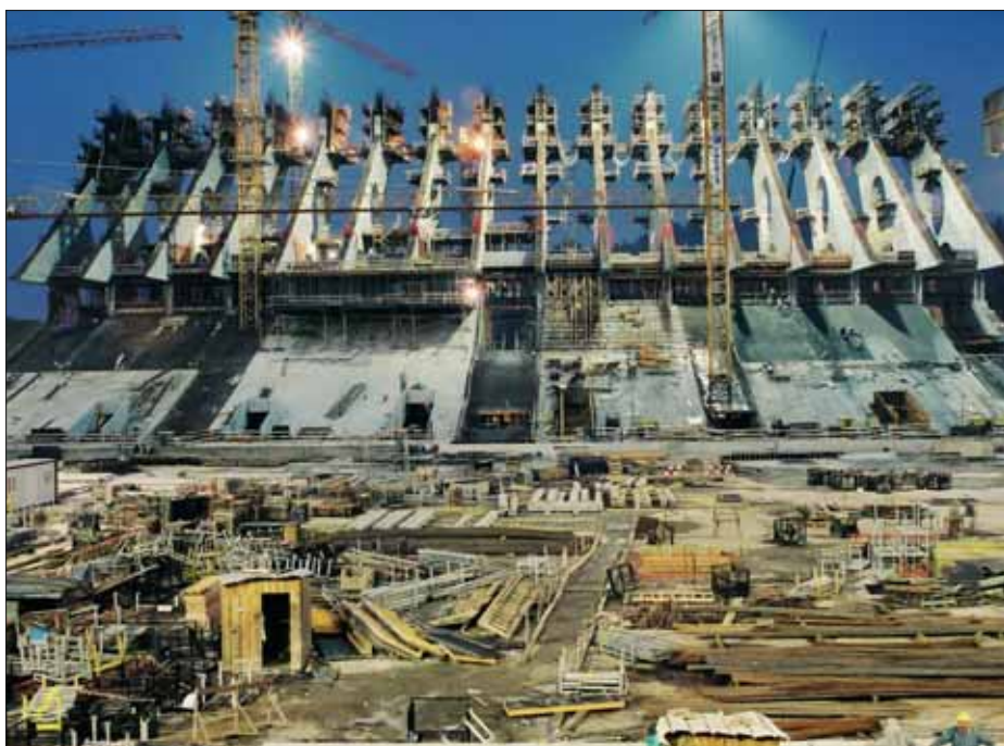
Fig. 7: East Stand during construction
