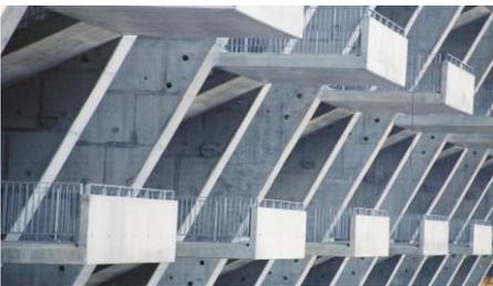
Visitors ascend the stand through stairs located between the uprights, which from level +110 onwards, have plinths placed at the intermediate levels (protruding from the uprights). There are also two panoramic lifts to transport loads and people between level +98 and level +112. The hydraulic and electrical infrastructures are placed inside the uprights and the slabs, from the level of the foundation to the level of the roof.
