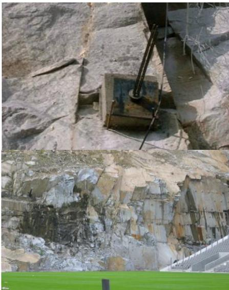
The west embankment, much smaller than the east one, was far easier to stabilise as the slope of the family of fractures was favourable. This embankment was also stabilised through anchoring and bolting.
