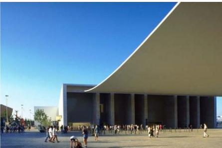
A suspended roof such as Siza's / ARUP/ STA'S Portuguese Pavilion in EXPO 98 came up as the natural solution. The rock was there to anchor the cables and the reaction of the roof in the cantilevered stand would "help" stabilising it. The doubt was the dynamic behaviour of a 220m span roof and the fact that the roof would have to be built 50m high (the Portuguese Pavilion is 67.5 m span and had been built with a total propping system from the ground!)
