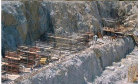
Preliminary information collected in the available resources and a preliminary geotechnical survey released our main worries: we would find the granite all way long but we would have to adapt the slopes to the level and orientation of the slipping plans of the rock, still to be determined. Time wouldn't be a problem if the excavation could begin and the cost of the excavation could be significantly reduced by selling the excavated material. In August 2000 the excavation contract began.
