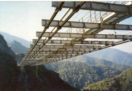
Research on similar structures and preliminary calculations showed the feasibility of the solution and that an appropriate geometry and slab weight could lead to a desirable balance of moments in the foundation for permanent combinations of loads.
