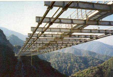
Research on similar structures and preliminary calculations showed the feasibility of the solution and that an appropriate geometry and slab weight could lead to a desirable balance of moments in the foundation for permanent combinations of loads.
