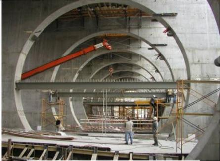
Structurally the East Stand functions without any dilation joint. Therefore the set of the 16 uprights with the slabs of the floors and the stands stabilise the structure of this stand in relation to both vertical and horizontal actions.
