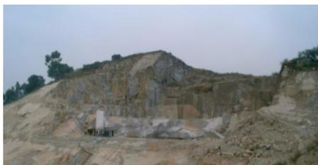
There was little geotechnical information available but the visible rock on the quarry gave us confidence to explore the route. The question was to know if we could trust that the rock was there in depth, and how would it stand in near vertical 50m high slopes. How much time would it take to excavate it and how much would it cost? We were in the beginning of 2000 and the Stadium should be finished by the end of 2003.
