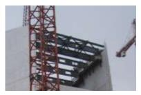
Given the slight slope of the roof panels, certain free edges which were to be very slender would have had excessive deformations unless the reinforced concrete shell had not been substituted by metallic structures comprised of open-web girders or beams in a welded, variable cross section construction. The rigidness of these edges is crucial in those situations where they support the glass panels of the large openings.
