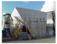
We should note that the compaction necessary to obtain the finishing and wall effect wanted meant that the white concrete used on the job had strength characteristics close to that of a C50/C60 concrete, much higher than the structural or durability requirements.
