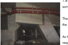
The pillars are circular with truncated conical shear heads and they are generally set out in a rectangular 7.8 x 7.8 m<sup>2</sup> grid. The vertical walls, in addition to being vertical support elements, also act as fire-walls, and sometimes they also act as support for the access ramps.
