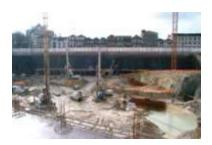
In the auditorium building, indirect foundations of piles sunk in slightly altered granite were used. In the car park, footings based in the gravelly layer present at the pillar base level were used.
