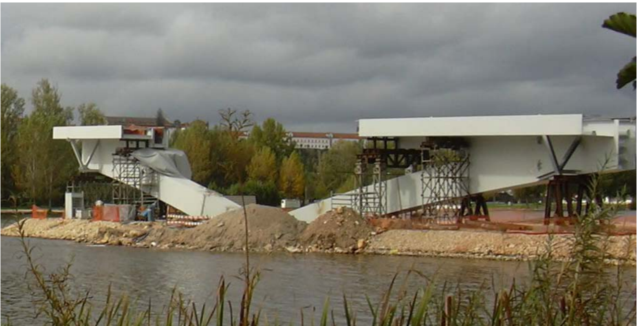
Fig. 6 – Details of propping of the bridge under construction (October 2005).
