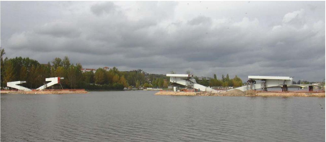
Fig. 6 – Bridge under construction (October 2005).
